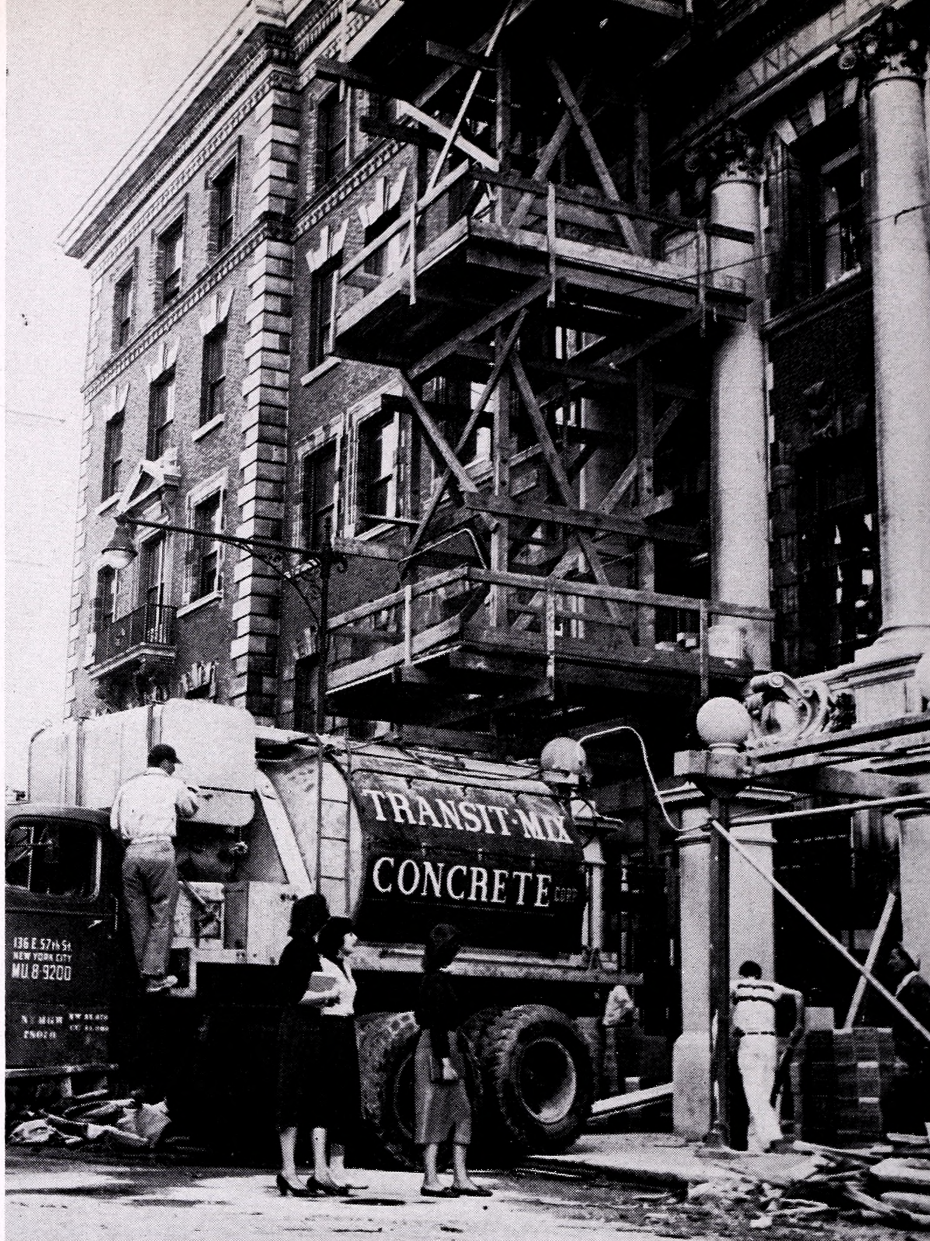
Returning students find Milbank still scaffolded and under repair
