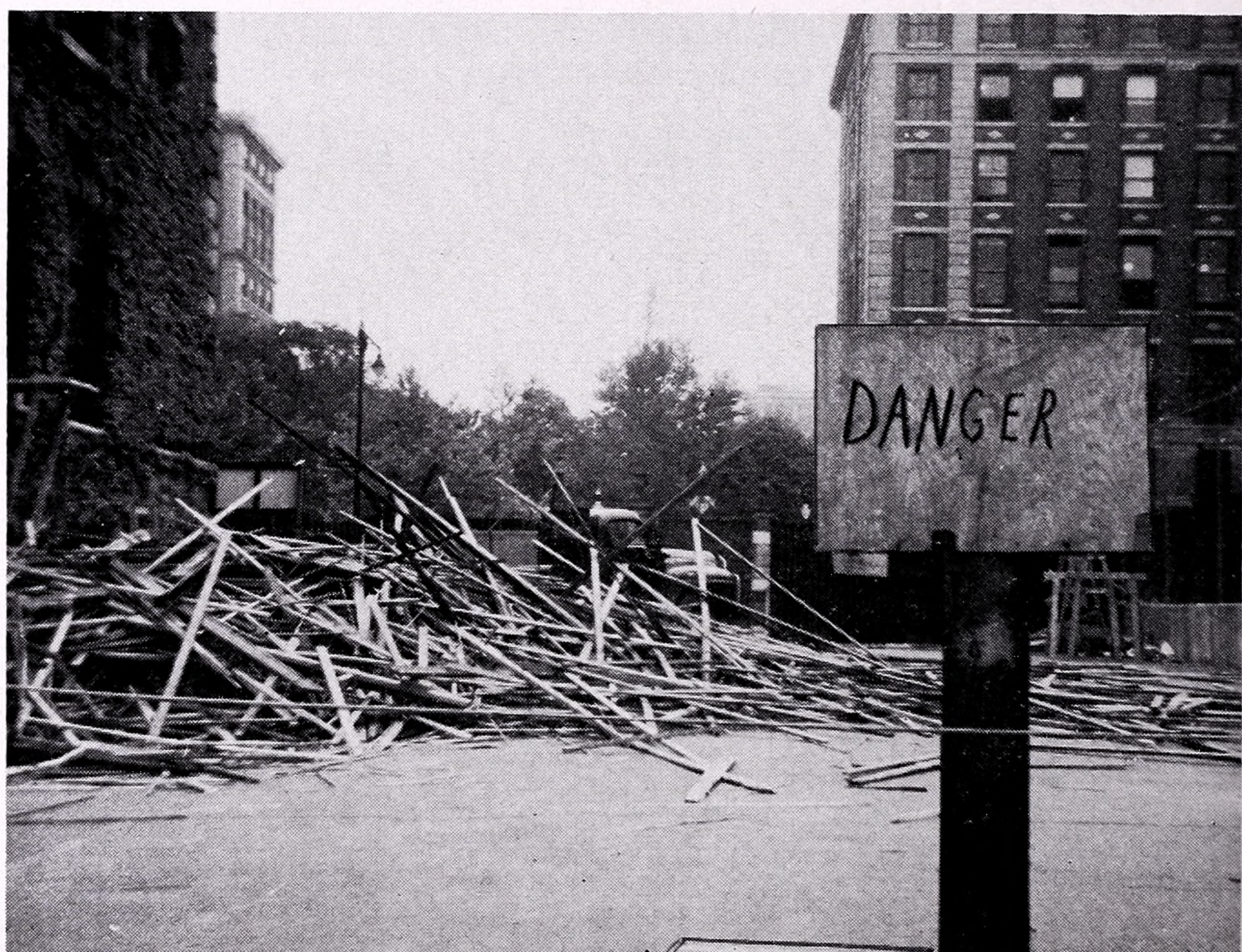
Old boards and other debris make crossing 119th Street a hazard
