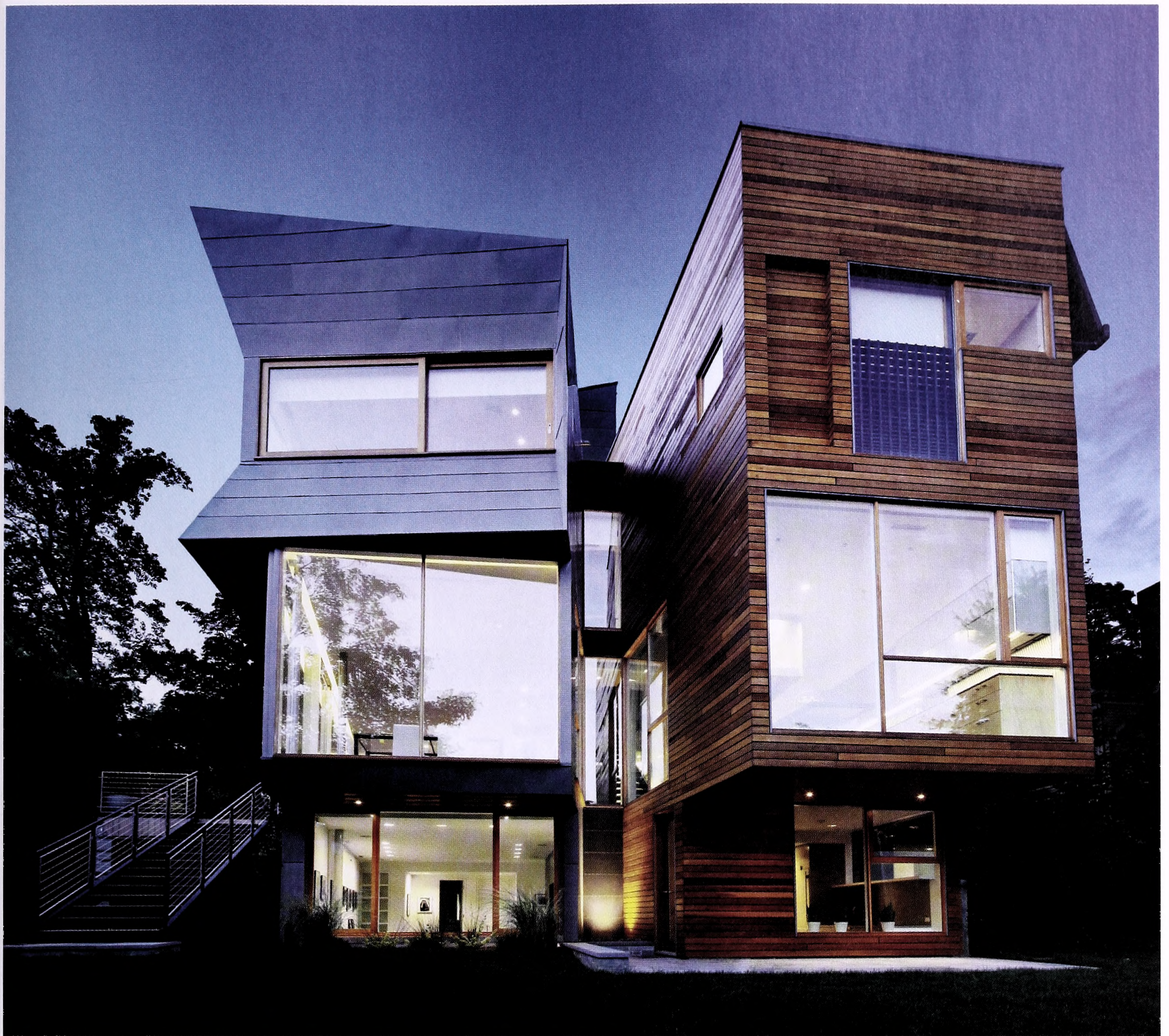
The rear-facade of the Town-House in New Canaan, Connecticut, by Joeb Moore + Partners. The structure is clad in zinc-coated copper and red-cedar siding.
