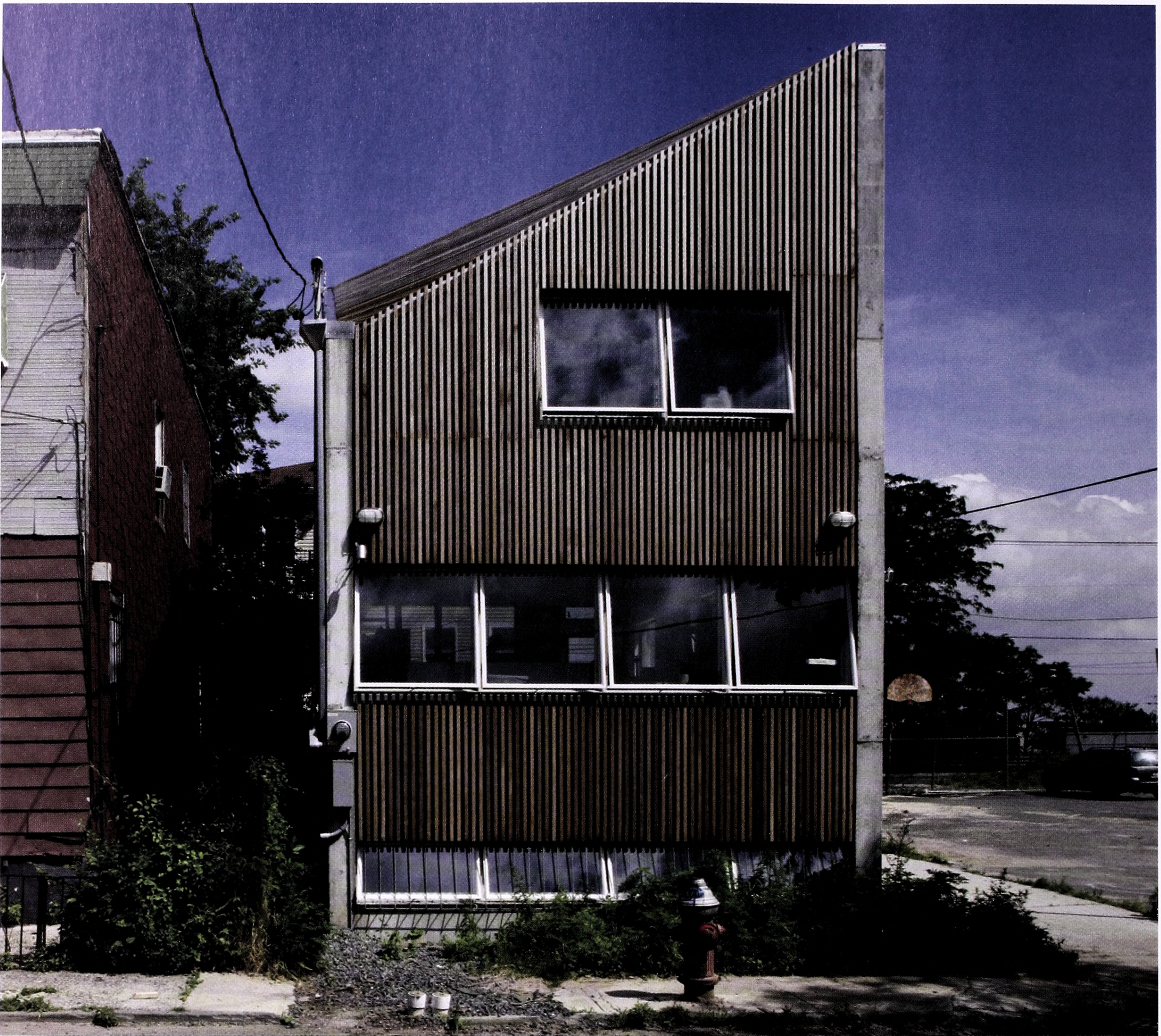
PREttyFAB house in Jersey City, New Jersey by GRO Architects. Pre-cast insulated concrete clad in cedar slats on the front facade. Photographs above and opposite, by Fabian Birgfeld, photoTECHTONICS
