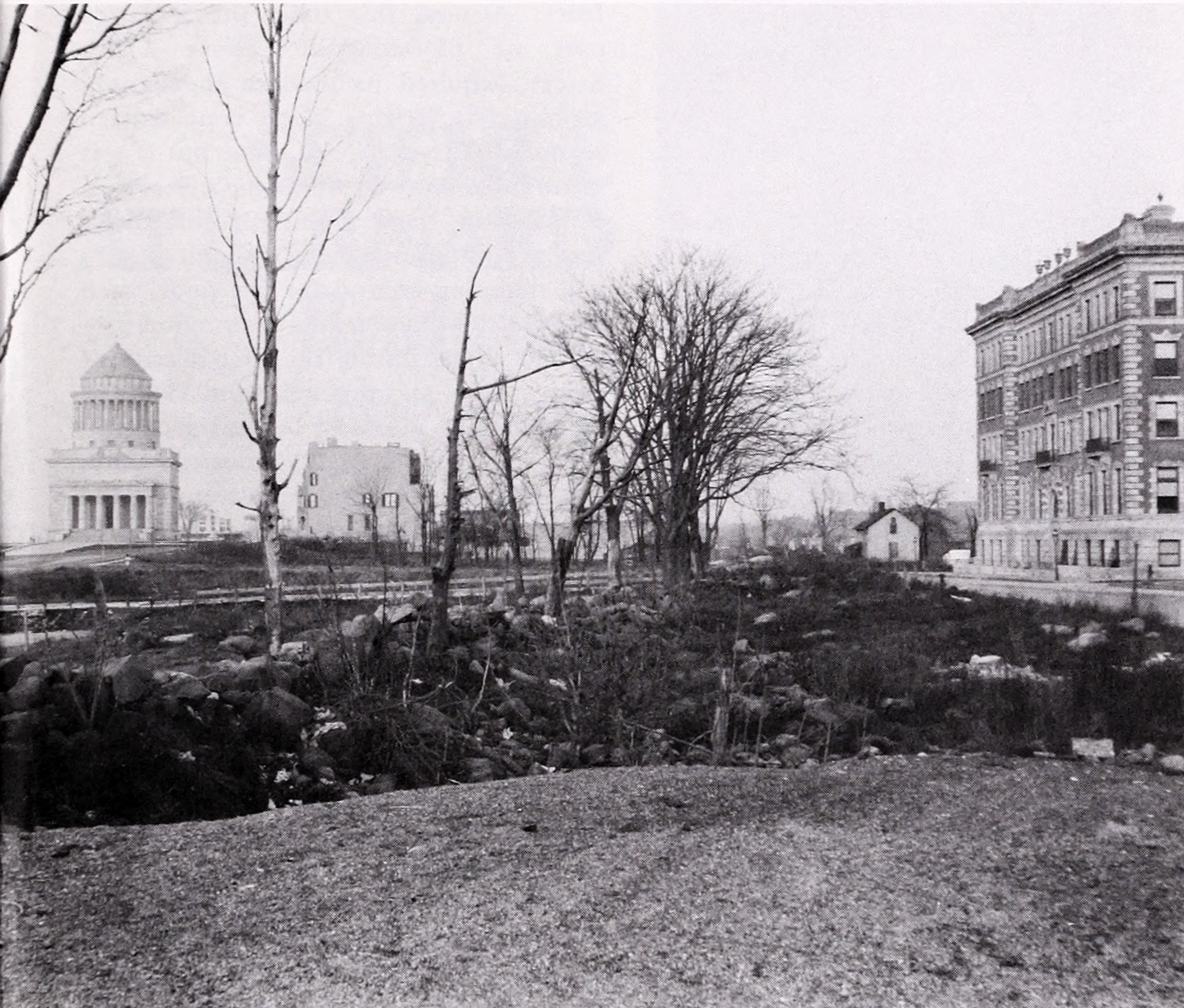
Bloomington Road in 1903, looking north from West 117th Street, west of Claremont Avenue. Note the farmhouse north of Milbank Hall.
