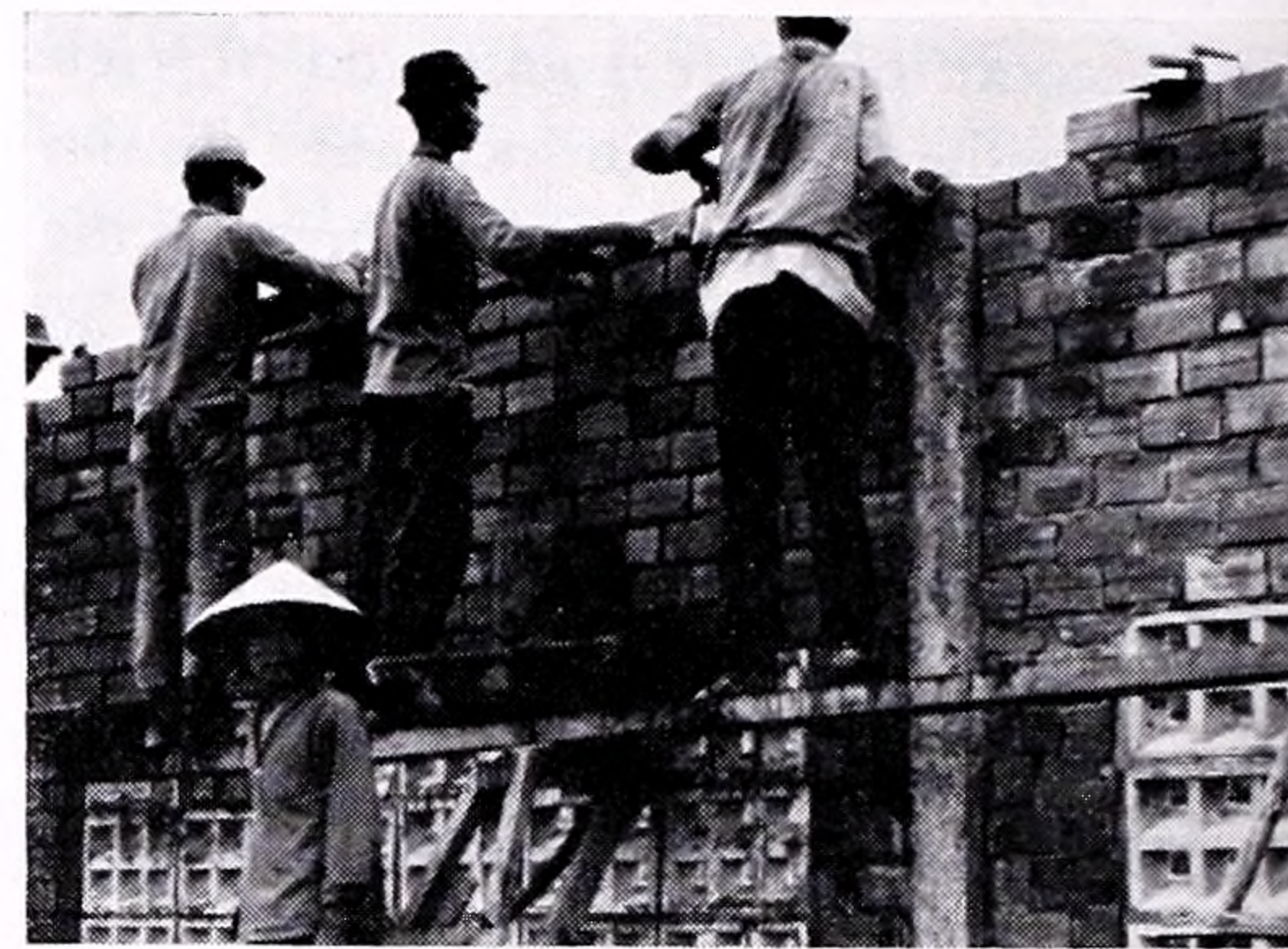
Building a school
