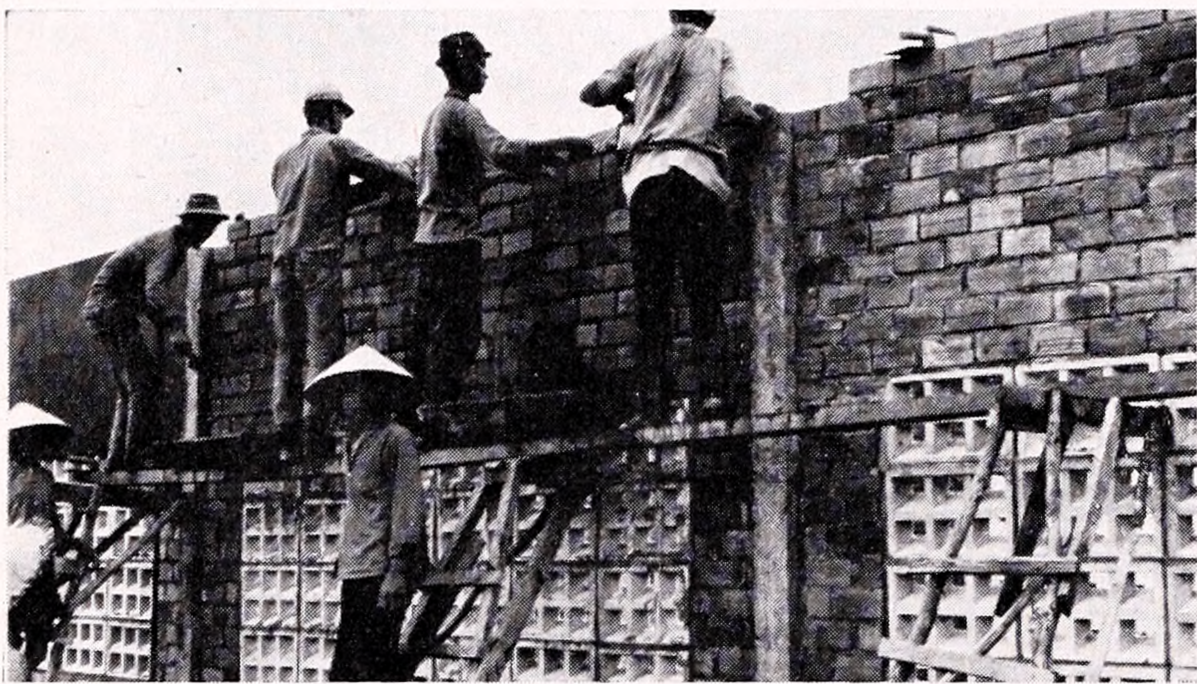
School building with U.S.-supplied cement
