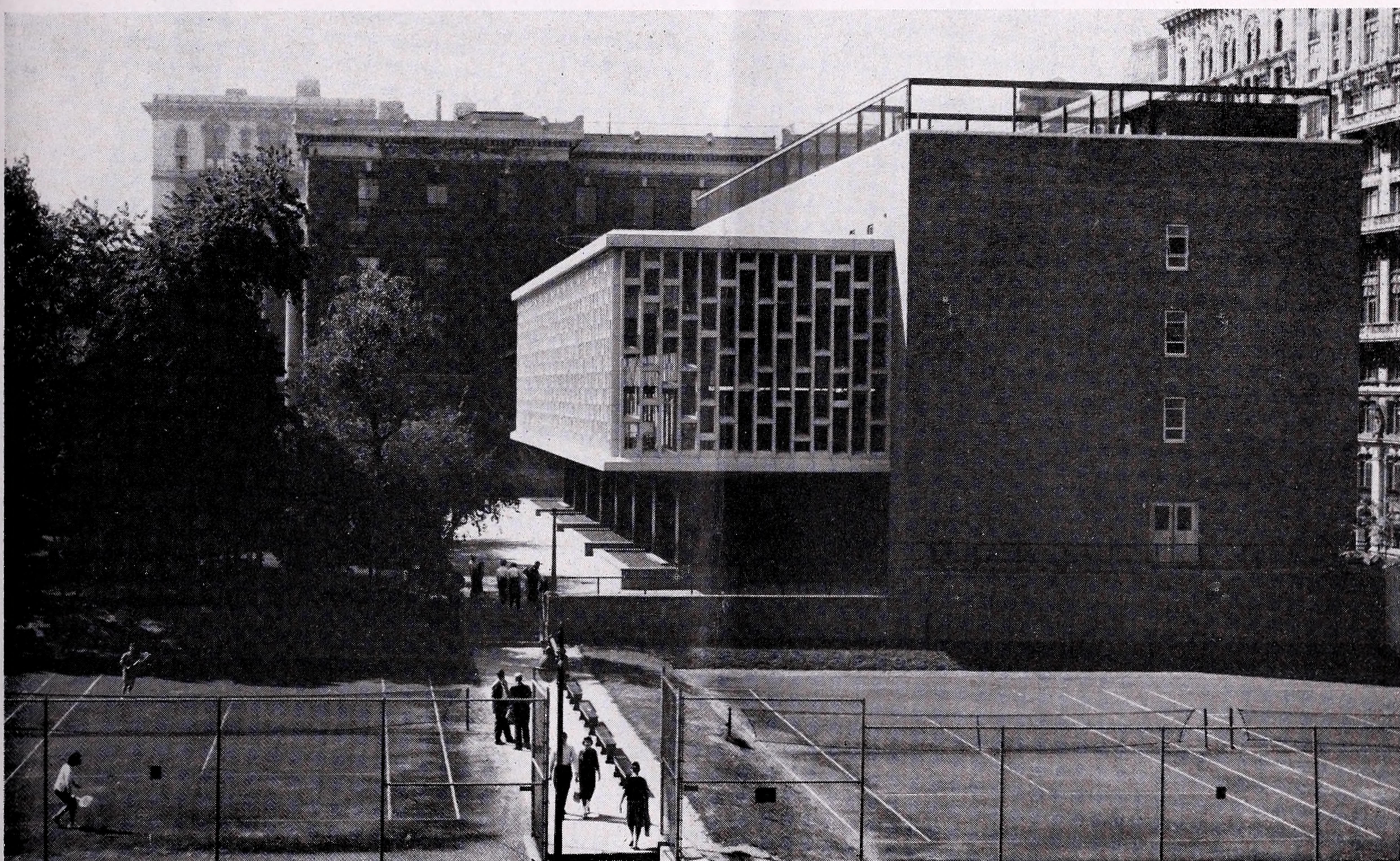
View to the south from Milbank Hall: red brick covers most of the building, relating it to others on campus. Second and third floors, walled by terra cotta and glass, jut out thirty-five feet in front. Tennis courts in foreground of photograph have partners on roof of new building, also containing archery range
