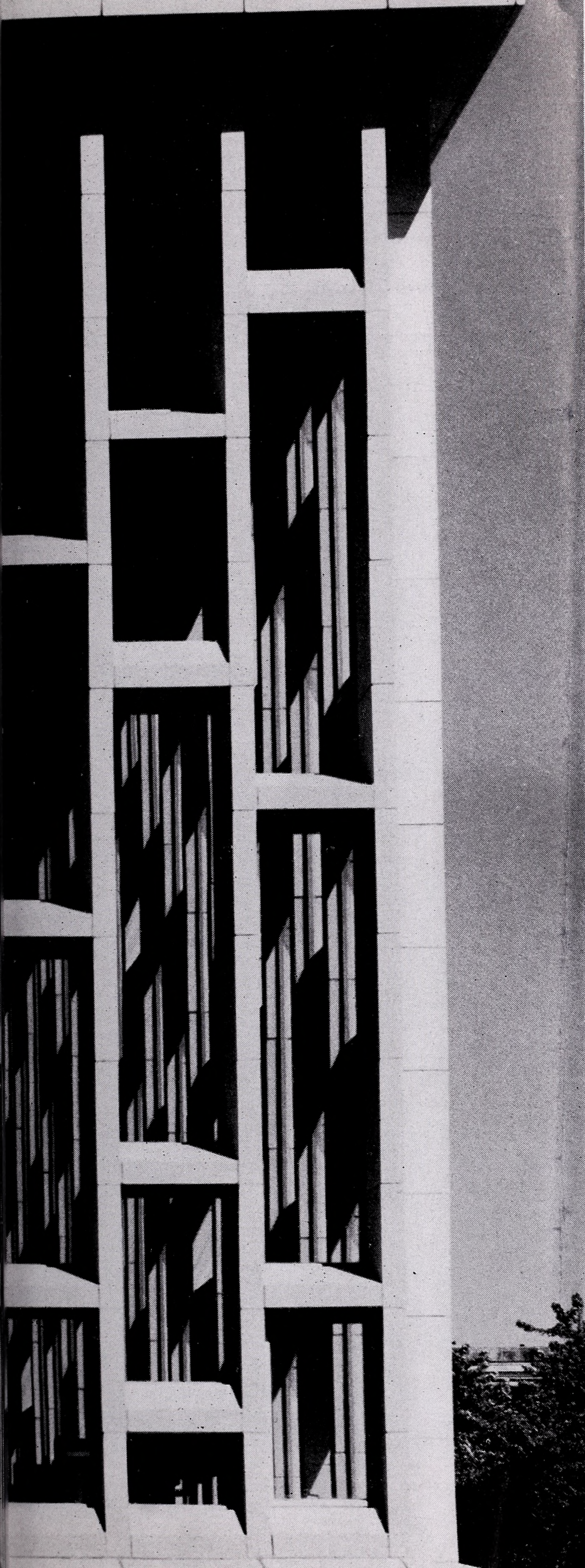
close-up view of library's glass and terra cotta facade by Rollie McKenna
