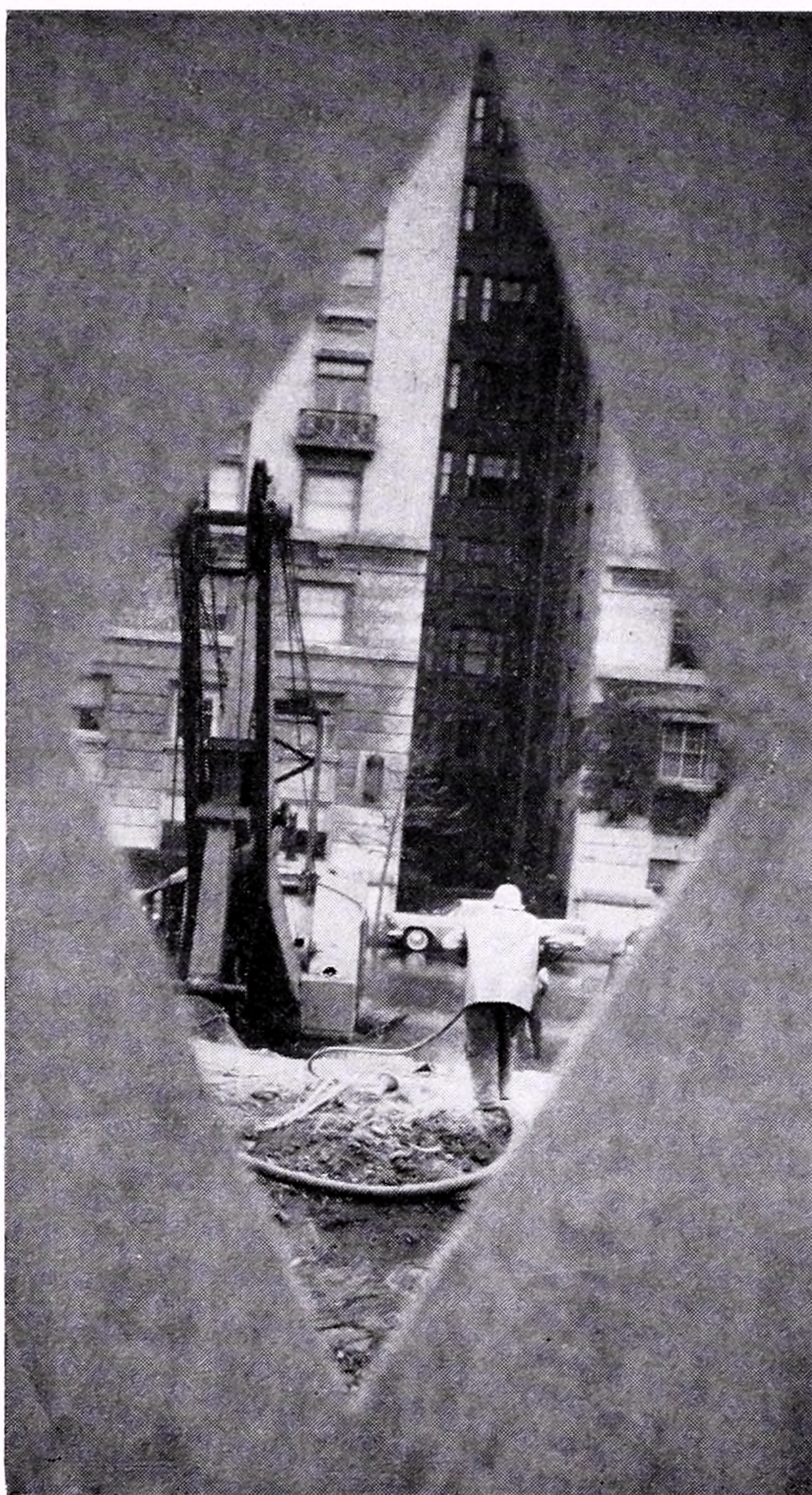
Construction underway on library building
