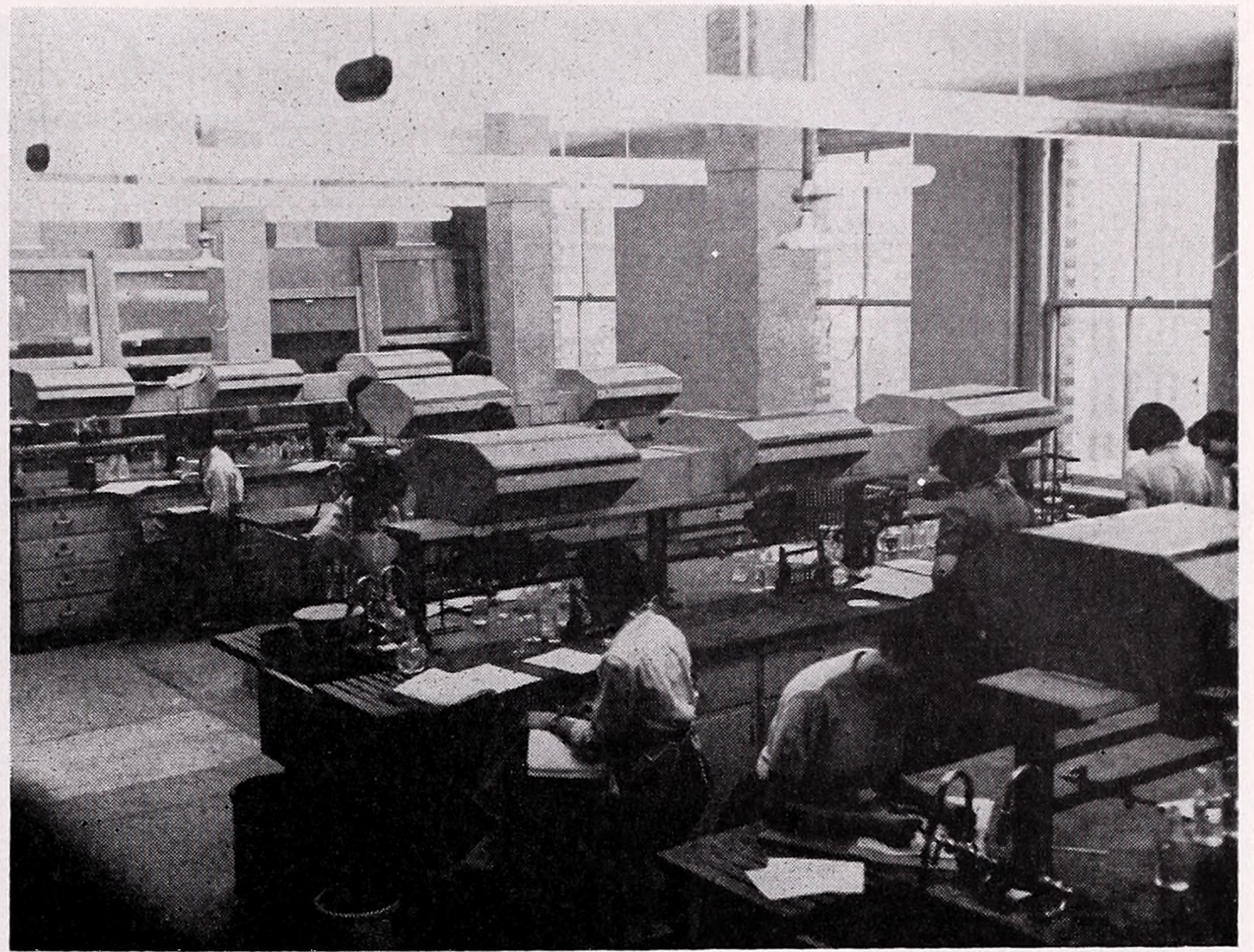
Renovating outmoded laboratories was major feature of rebuilding; typical of improvements in other science departments are new lights and modern work tables in elementary chemistry class's laboratory
